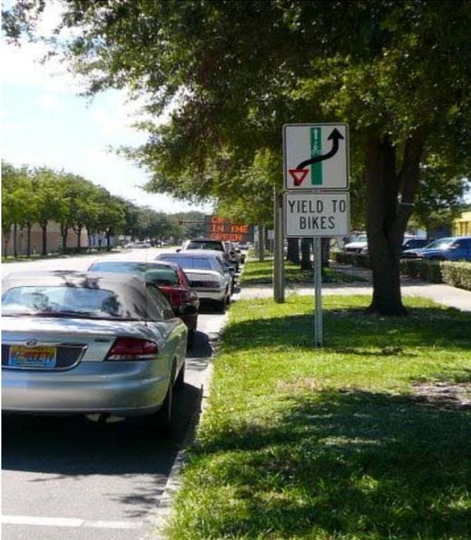
**Figure 3. Sign assembly used in the vicinity of the green bike lane weaving area.**
