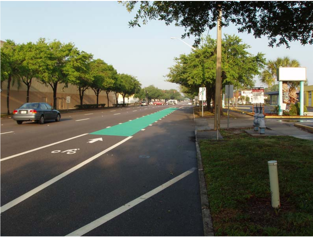
Figure 2. First “after” condition for green bike lane weaving area.
