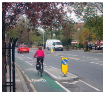
Maintain cycle lane width past separations
