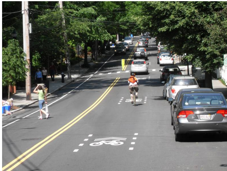
Figure 5: Bicycle priority lanes on Longwood Avenue in Brookline, MA. The bracketed sharrow modules are 5 ft wide and 20 ft long, with an 80 ft gap between modules.
