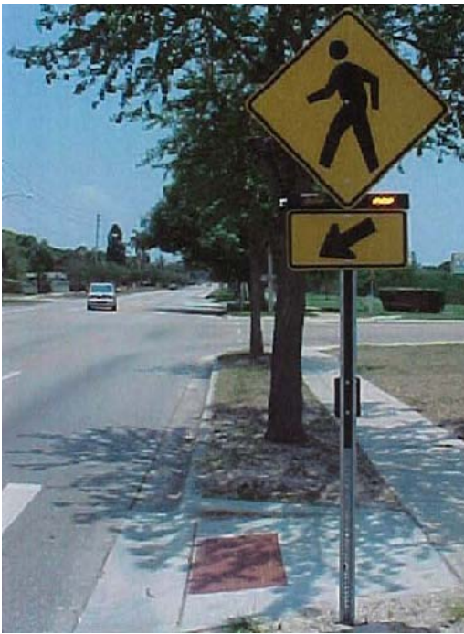
Example of RRFB with W11-2 sign and W16-7p plaque at crosswalk across uncontrolled approach. [Photo courtesy of City of St. Petersburg, Florida]
