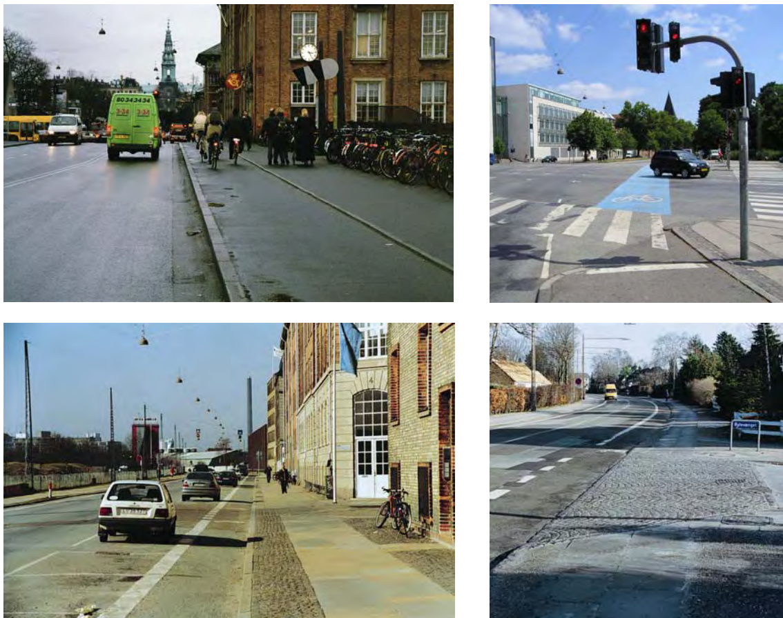
Figure 1. Photos of cycle track (top left), cycle lane (bottom left), blue cycle crossing (top right) and raised exit (bottom right).
