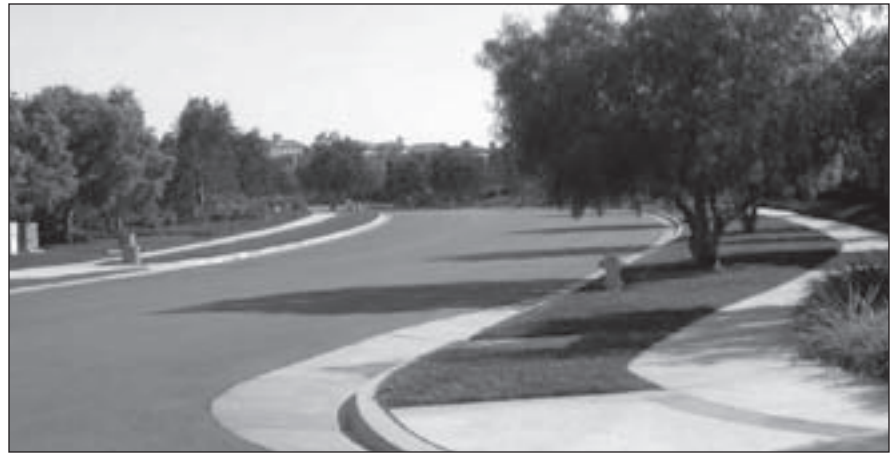
Figure 4. Chambord Road before restriping.
