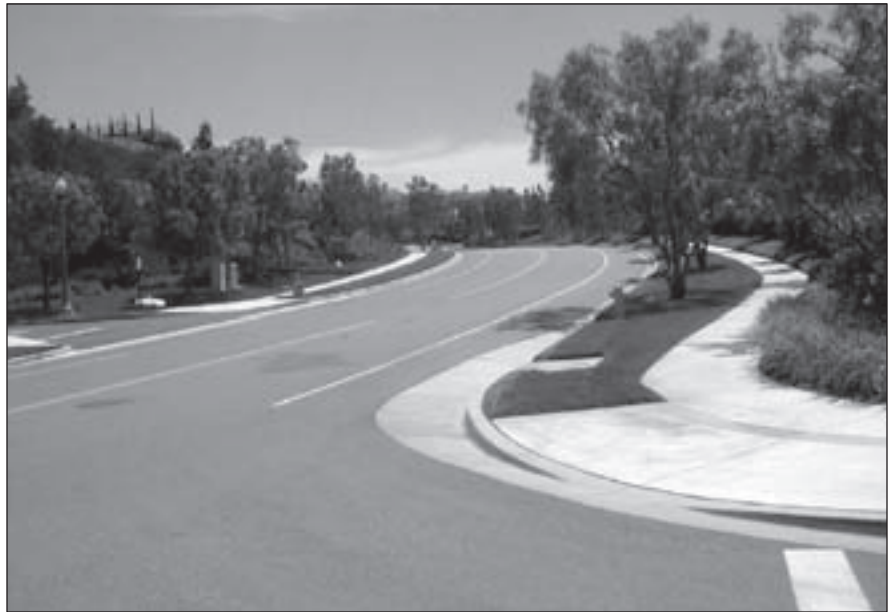
Figure 1. Typical traffic calming striping.
