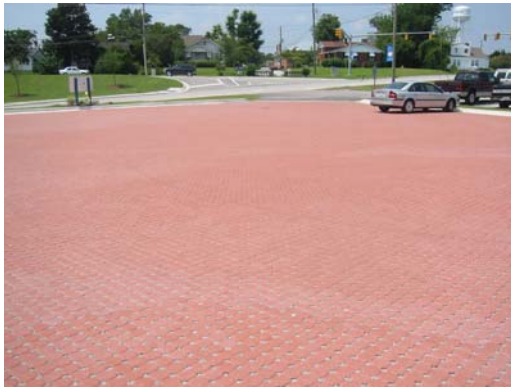
Figures 5a and 5b. Swansboro monitoring site and close up of PICP at the site.
