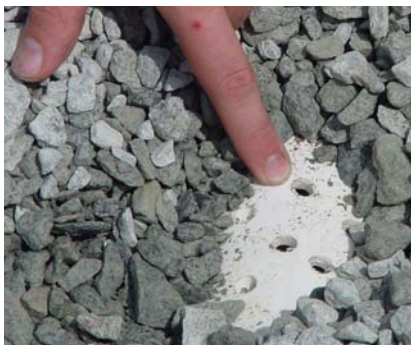
Figure 4. PVC drainpipe with infiltrate holes installed under PICP in stone layer at the Goldsboro site.
