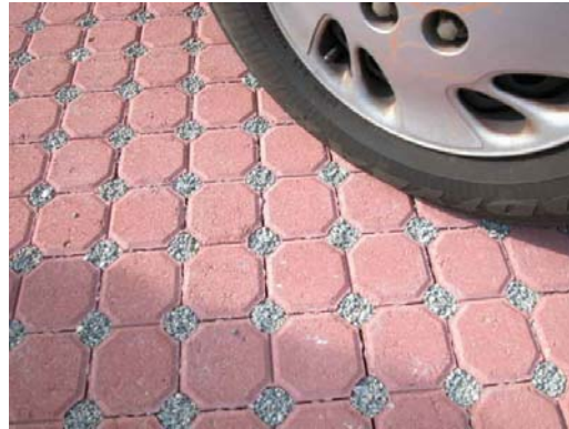
Figures 5a and 5b. Swansboro monitoring site and close up of PICP at the site.
