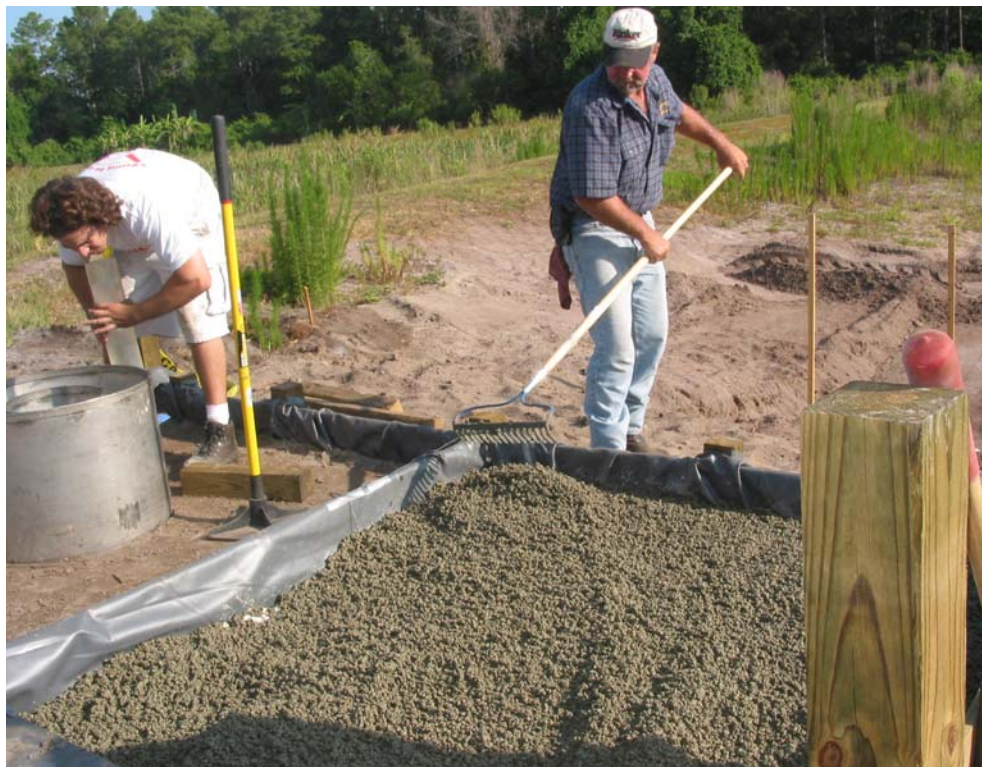
Figure 3: Stormwater Academy Porous Concrete Test Cell Installation
