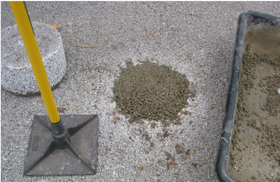
Figure 11: Repair of Concrete Core Area
