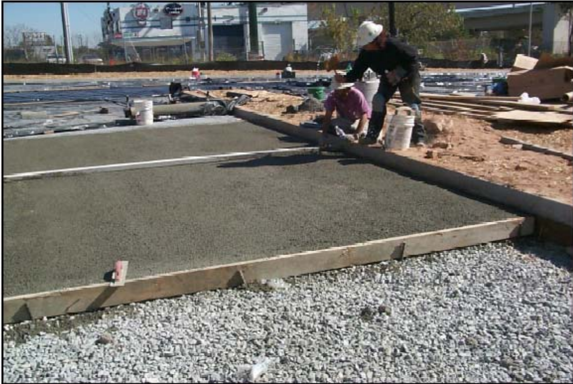
Figure 2: Typical Porous Concrete Installation
