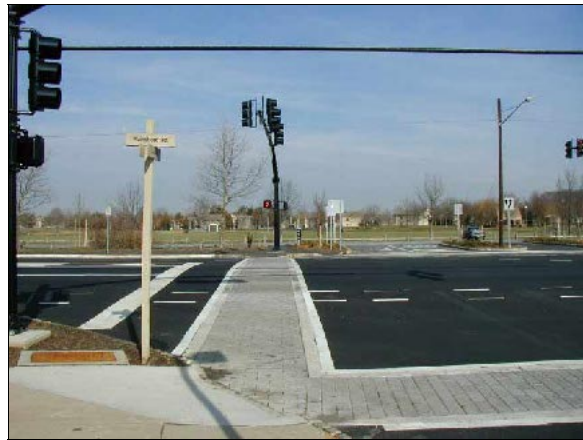
Figure 11: After - Signal, Stop Line and Bike Lanes
