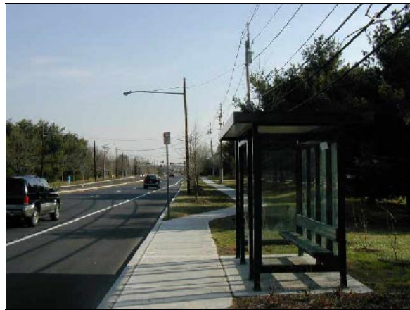
Figure 5: After – Curbs, Sidewalk, Bus Shelter, Street Trees
