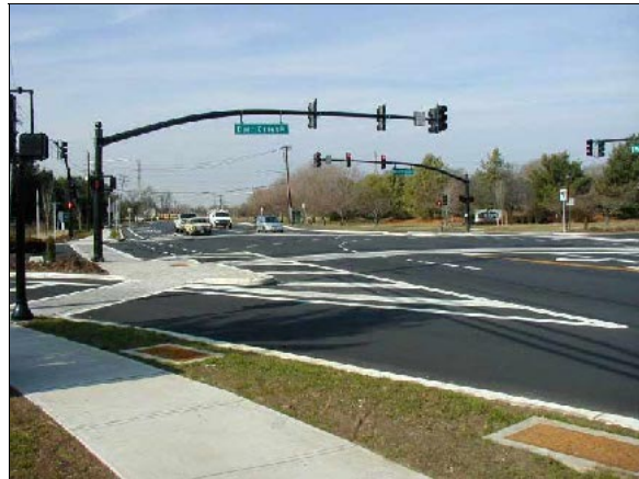
Figure 7: After – Signalized Intersection with Textured Crosswalks and Expanded Islands
