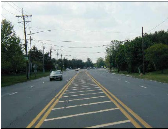
Figure 2: Before - Flush Median
