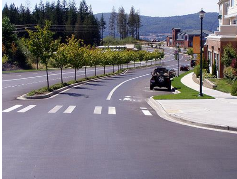
Figure 4 – A bar pair crosswalk that is spaced so as to avoid the wheel path of automobiles. (Source: Dan Burden, 2006. www.pedbikeimages.org )
