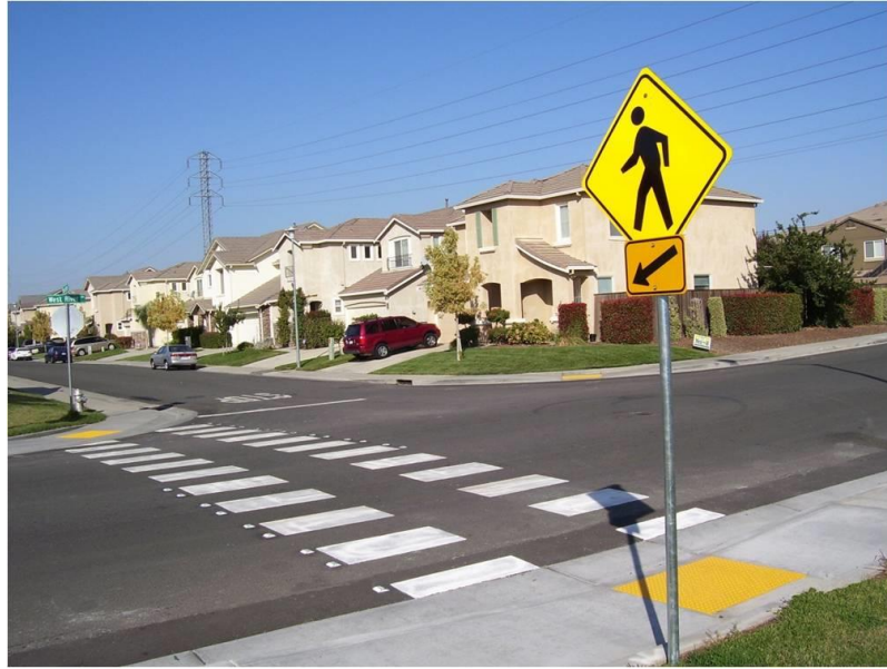
Figure 5 – A triple-four crosswalk pattern, which is the standard crosswalk style in Sacramento, CA. This pattern is high-visibility, has a center channel that is less slippery, and has bars spaced so as to reduce maintenance costs. (Source: City of Sacramento, http://www.cityofsacramento.org/transportation/dot_media/engineer_media/traffictriplefourcrosswalk.jpg )
