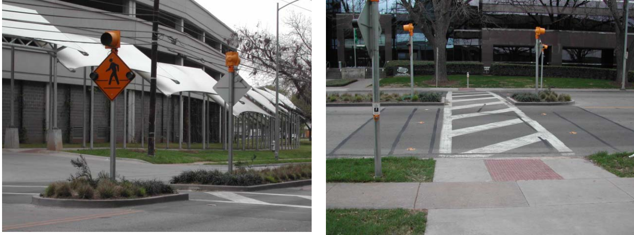
FIGURE 2 In-Roadway Warning Lights Treatment at Site 3.
