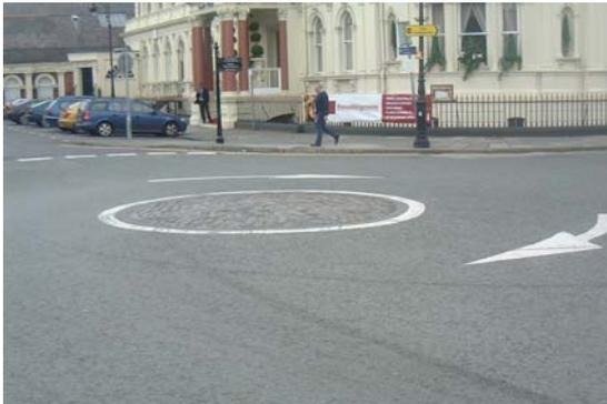
Photograph 6: Non-conforming central marking in setts with white edge marking
