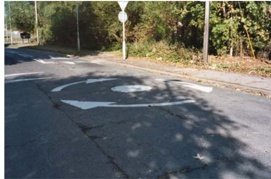
Photograph 8: Central island positioned so drivers have to pass over it to negotiate junction
