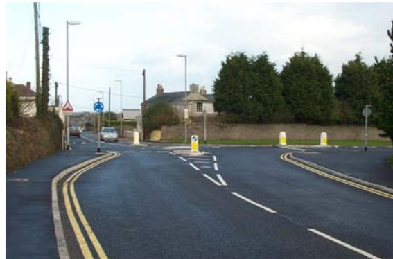
Photograph 10: Deflection through alignment and traffic island
