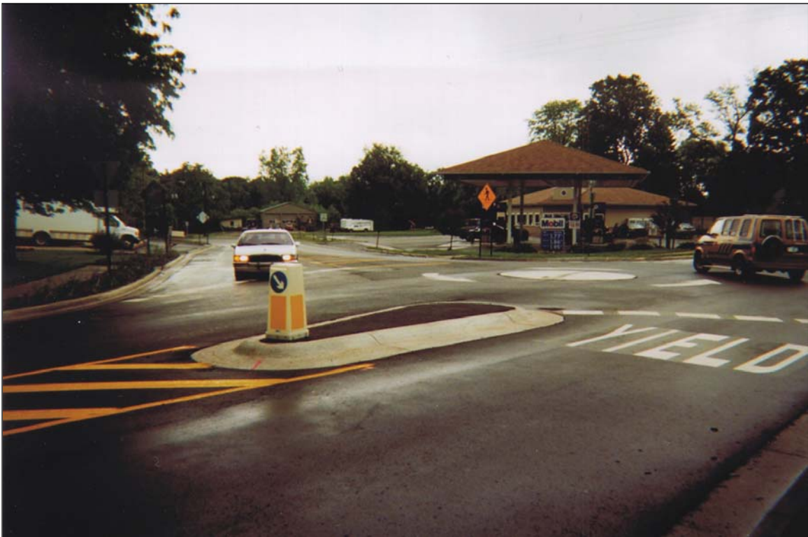
Figure 3 Looking Northeast at the Dimondale Mini-Roundabout
