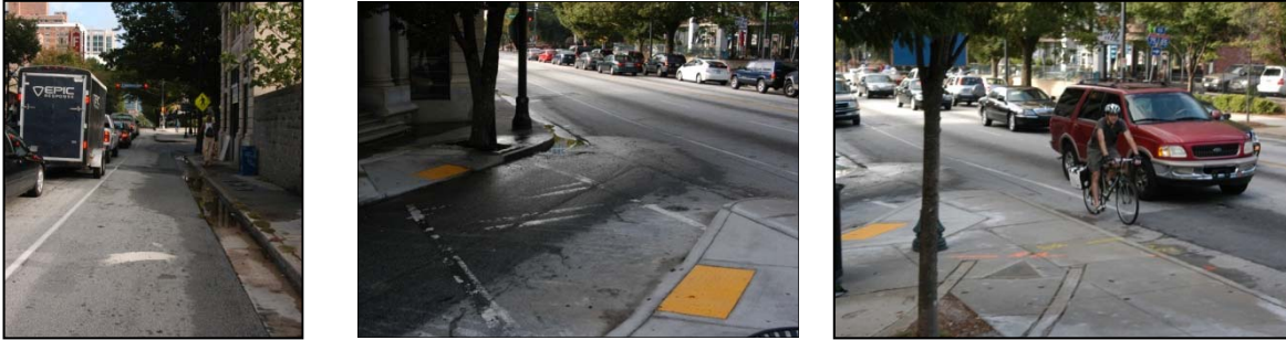
Incompatible right-turn channelization at the intersection of Peachtree Street and Ponce de Leon Avenue.
