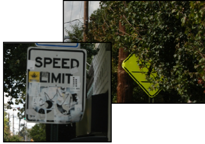
Signs along North Highland Avenue that were vandalized or blocked by trees.
