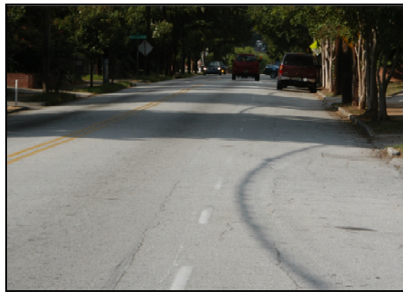
A portion of North Highland Avenue that transitions from two travel lanes to one travel lane and on-street parking.
