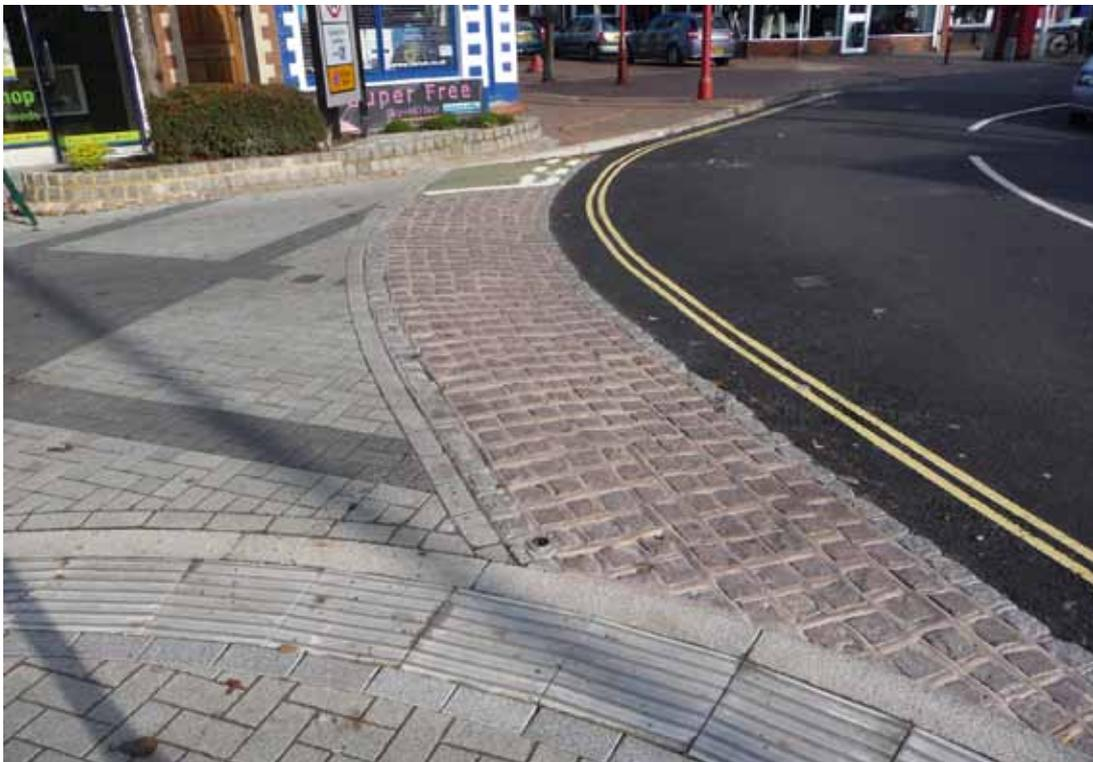
Figure 6.2 Example of a shared space gateway feature
