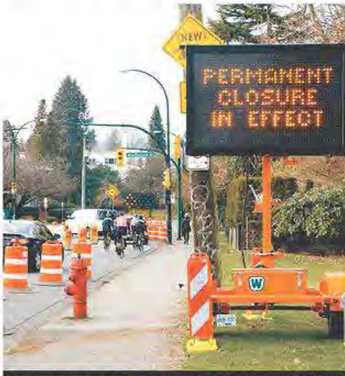
Concrete barriers and pylons block through traffic for cars on Point Grey Road from Macdonald to Alma streets. EMILY JACKSON/METRO
