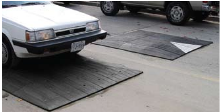
Speed cushions showing impact on typical vehicles: Vancouver, Canada (Credit: Richard Drdul) (Note: for illustrative purposes only)
