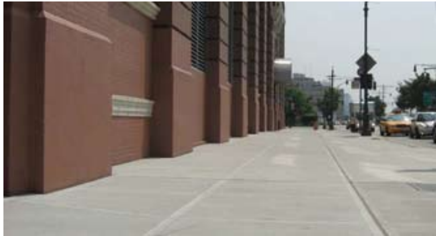
Typical concrete sidewalk: West Street at 16th Street, Manhattan
