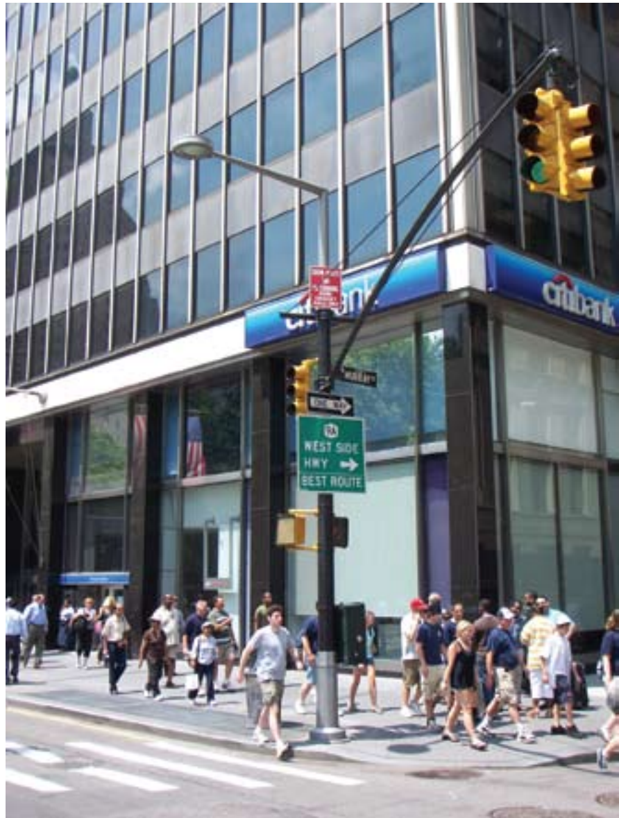
Alliance Traffic Signal Pole and luminaire: Murray Street, Manhattan
