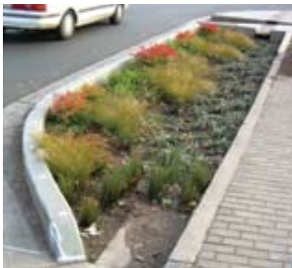
Curb extension with a planted swale that captures stormwater from the gutter: Portland, OR (Credit: Abby Hall)
