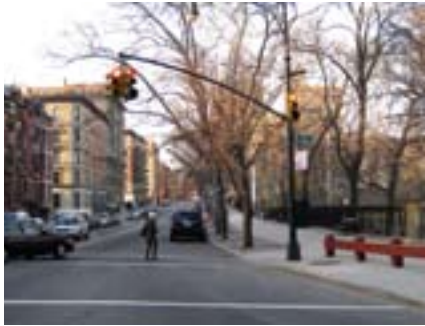
Type M-2 Traffic Signal Pole with historic luminaire: West 113th Street, Manhattan
