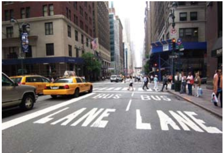
Curb-aligned double bus lane: Madison Avenue, Manhattan
