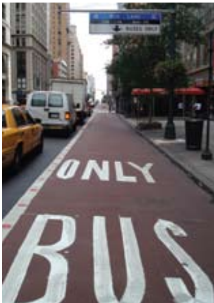
Red, curb-aligned, on-street busway with "soft separation" from traffic: 34th Street, Manhattan
