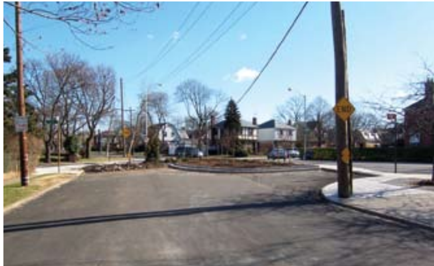
Full closure with Greenstreet and turnaround: Jewel Avenue, Queens
