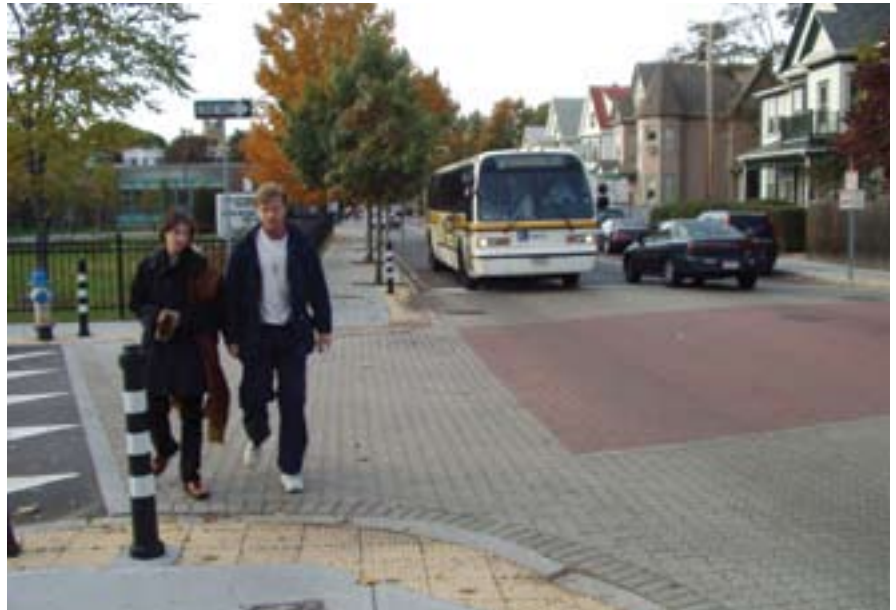
Raised Intersection: Cambridge, Massachusetts
