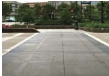
Long granite pavers set in poured concrete: West Side Highway, Manhattan
