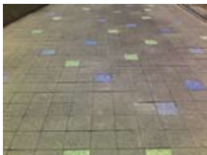
Concrete pavers with exposed blue and green glass aggregate (shown interspersed with black asphalt pavers): Hudson River Park, Manhattan
