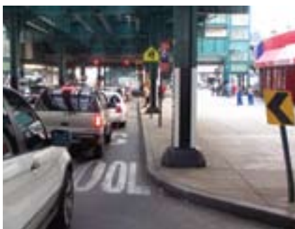
A bus bulb under an "El" (elevated subway): Jerome Avenue, The Bronx
