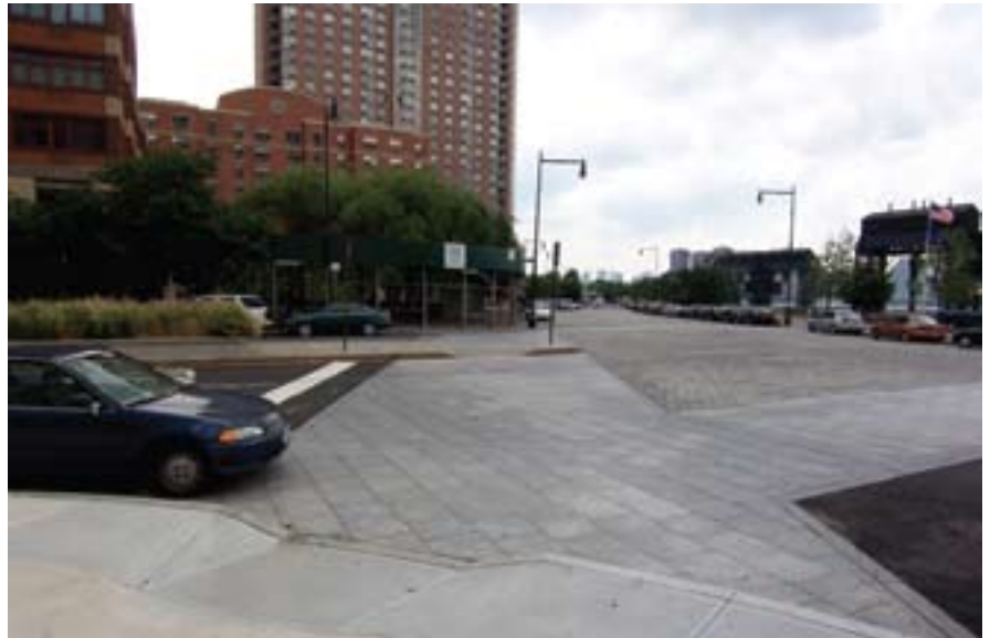
Example of square granite pavers in a crosswalk: 48th Avenue at Center Boulevard, Queens
