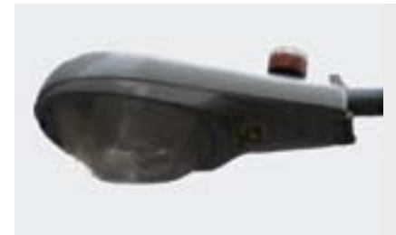
Cobra Head luminaire: Manhattan Bridge, Manhattan
