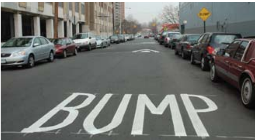
Speed hump: Bolton Avenue, The Bronx
