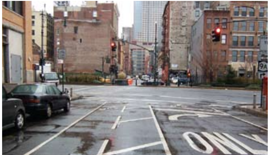
Median barrier: Canal Street, Manhattan
