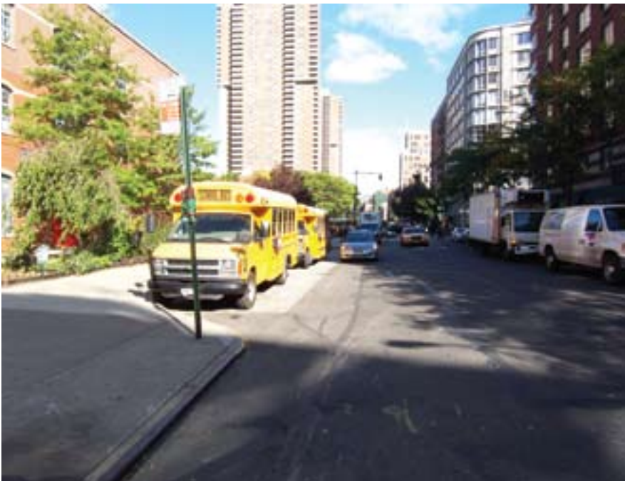
Lay-bys for curbside loading between curb extensions: Greenwich Street, Manhattan
