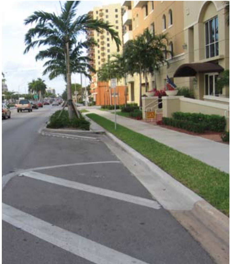
Precast concrete curb and gutter sections laid end-to-end. Photo shows optional sidewalk extension in background: Miami Beach, FL
