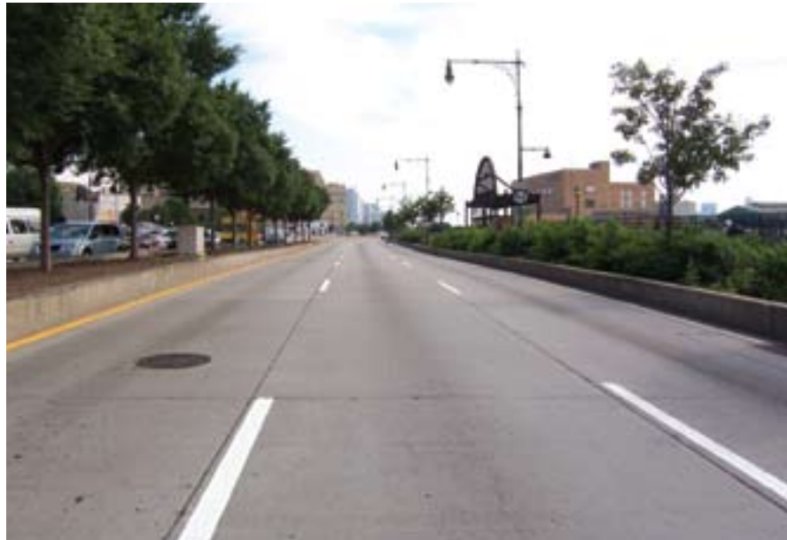
Typical concrete roadbed: West Side Highway, Manhattan
