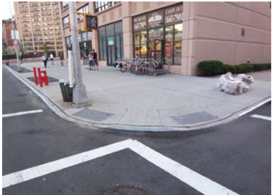
Sidewalk corner quadrant with pedestrian ramps: West 110th Street, Manhattan
