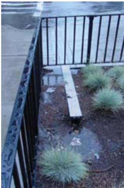
Detail of stormwater-capturing design during rain event (Credit: NYC DPR)
