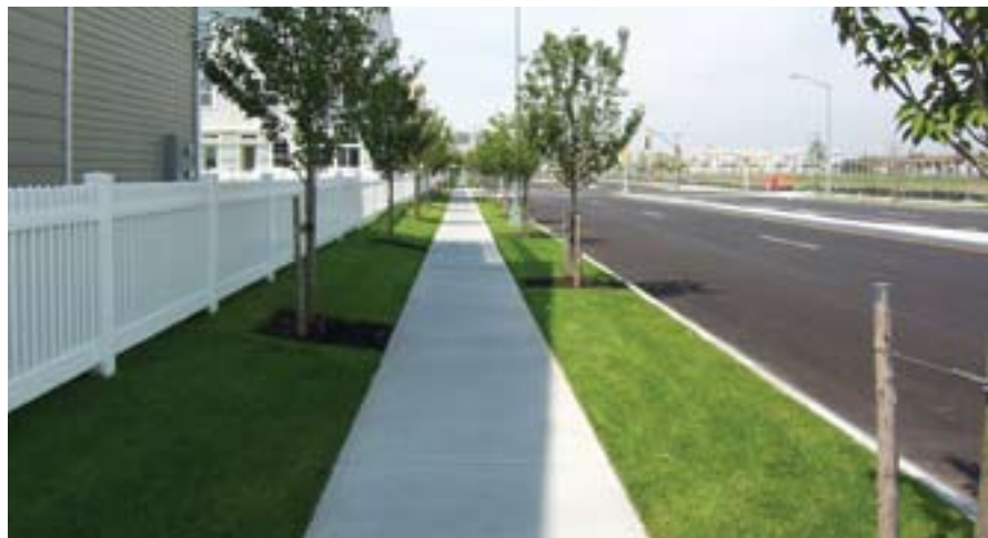
Concrete ribbon sidewalk: Rockaway Beach Boulevard, Queens
