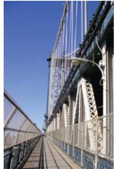
Cobra Head luminaire: Manhattan Bridge, Manhattan
