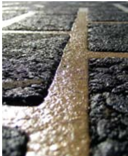
Close-up of thermoplastic imprinting: Seattle, WA (Credit: Integrated Paving Concepts)
