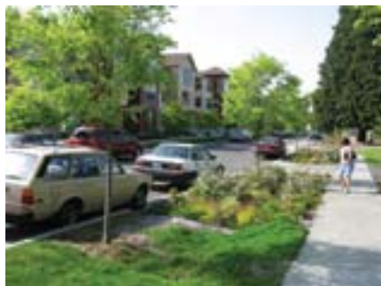
Ribbon sidewalk with Street Swale planting strip: Seattle, Washington (Credit: Abby Hall)
