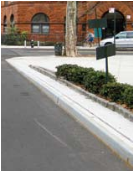
Typical untinted concrete curb with steel facing: West 114th Street and Morningside Avenue, Manhattan
