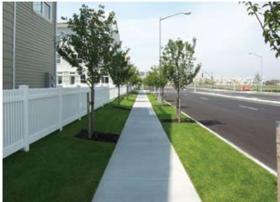
Ribbon sidewalk with lawn planting strip: Rockaway Beach Boulevard, Queens
