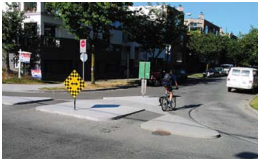
Forced turn with bike channel: Vancouver, Canada (Credit: Richard Drdul) (Note: for illustrative purposes only)
