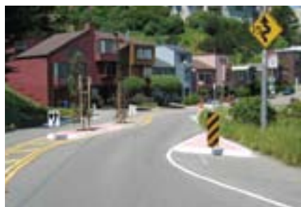
Chicane at entry to residential neighborhood: San Francisco, California (Credit: SF MTA)
