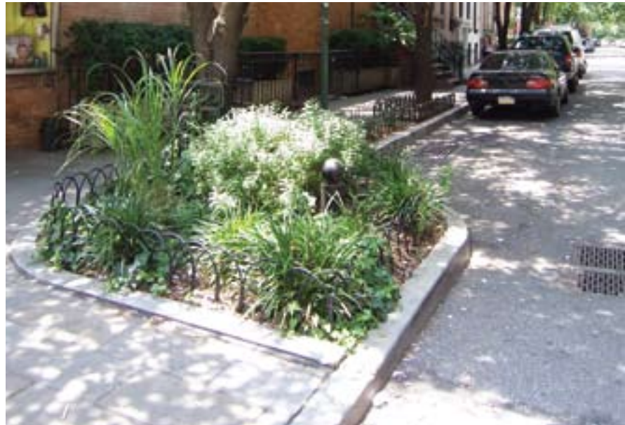
Curb extension with greenstreet: Mulry Square, Manhattan
