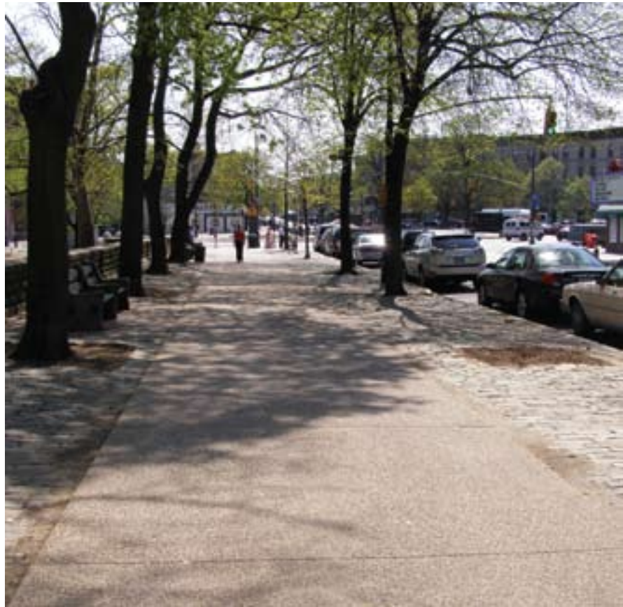
Sand-colored concrete sidewalk with exposed aggregate: Prospect Park West, Brooklyn
