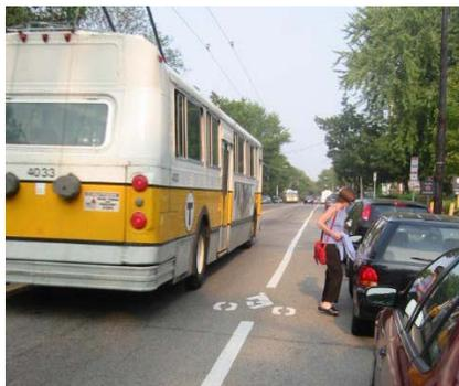
**Size/ Shape:** Bicycle stencil placed in a break of a continuous white line
